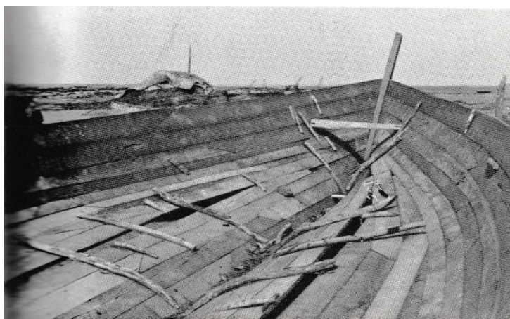
Figure 10 Almost finished planking of hora. It is shell without the frames inserted for strengthening. (Greenhill 1971)
